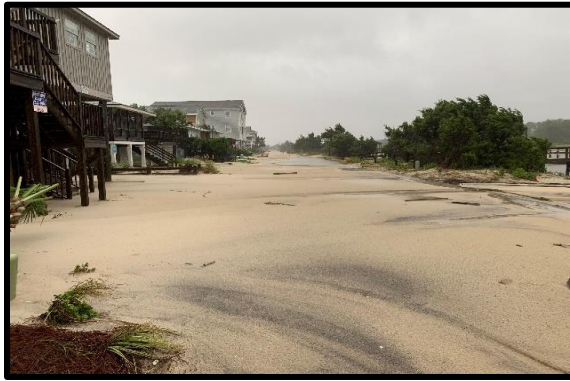
Figure 14: Springs Avenue After Hurricane Dorian (2019)
