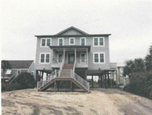
FRONT (ROAD SIDE)
